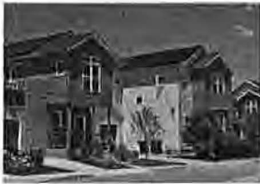
Figure 4. A solar subdivision in Boulder includes IPS solar installations. Photo from MRG & Associates
