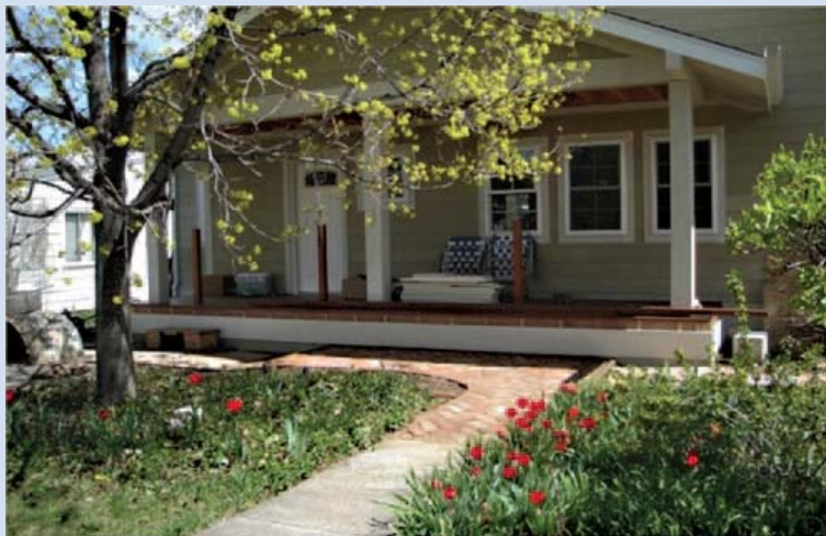
The Flax home is a demonstration project, using the ClimateSmart program as a starting point for developing livable, sustainable smaller homes. Photo from MRG & Associates
