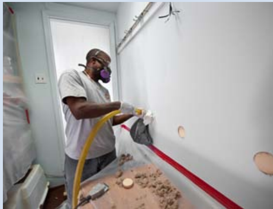
Photo by Dennis Schroeder, NREL/PIX 17963
