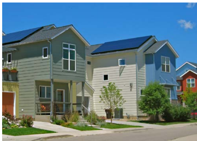
Figure 4. A solar subdivision in Boulder includes IPS solar installations. Photo from MRG & Associates
