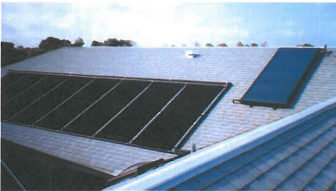
This photo shows two other non-PV solar collector types, a solar pool heater in the bottom left and a solar domestic hot water heater in the upper right. Although the solar water heater in the upper right may look similar to the PV modules in the grid tied example, the copper tubing extending off the upper right and bottom left of the collector indicates that these are hot water collectors. (Photo Credit – The Leveredge)
