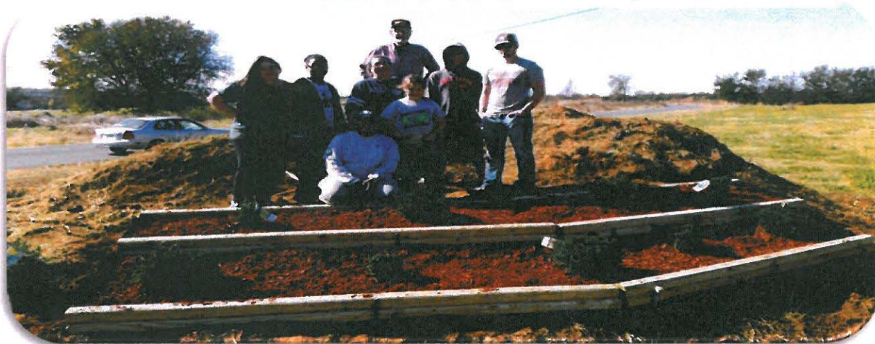
Phase I of the project completed. November 8, 2014
