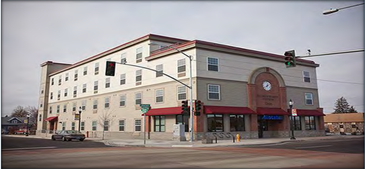
AHP funding will be used to rehabilitate vacant commercial building Market Street Station in Spokane, Washington, into a 33-unit apartment building for seniors age 55 and older, for households with disabilities, and for formerly homeless individuals. The building also will include commercial space.
