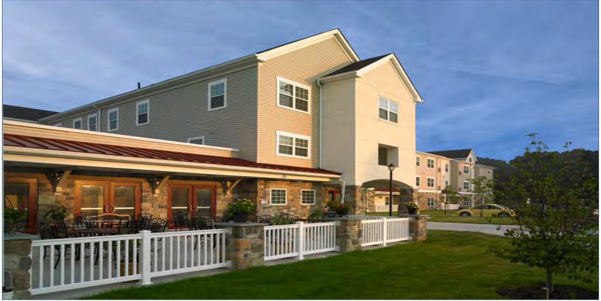
The Borough of Elverson, Pennsylvania, recycled a firehouse and transformed it into a 71-unit rental development for seniors using AHP funds.
